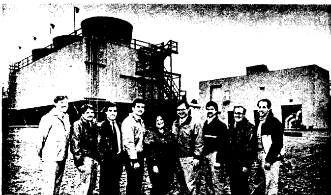
Behind the Central Chilled Water Facility and its cooling tower are some of those who worked on the project: (from left) Walter Bay, Plant Engineering Division (PE); Kenneth Davis, PE; Michael Furey, Division of Contracts & Procurement; Martin Fallier, PE; Marilyn Gibbons, PE; Edward Murphy, PE; Paul Coleman, PE; Mark Culp, PE; and Thomas Nehring, PE.
