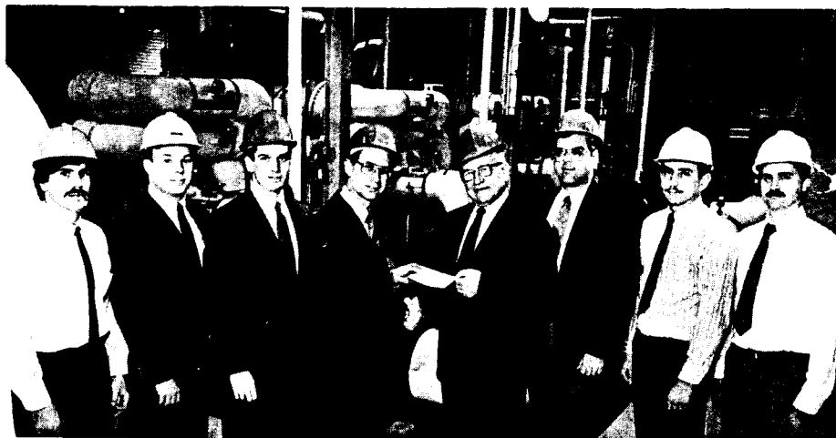
After BNL demonstrated operation of the Central Chilled Water Facility to the Long Island Lighting Company, a check for $400,000 was passed from LILCO Vice President Edward Youngling (center, left), of LILCO's Office of Conservation and Load Management, to BNL's Associate Director for Management and Physical Plant Parke Rohrer (center, right). The hand-off came as a result of BNL's participation in LILCO's "Dollars and Sense" program. Witnessing the rebate were: (from left) Mark Toscano, BNL's Plant Engineering Division (PE); Edward Murphy, PE; Philip Austen, LILCO; PE Manager Michael Bebon; Martin Fallier, PE; and Paul Coleman, PE. Behind the group are the three electric chillers.
