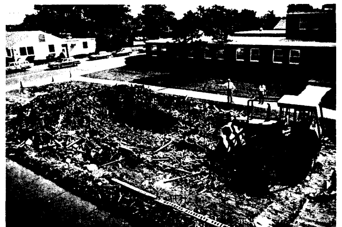
As the bulldozer dispenses with the remains of Bldg. 178, Parke Rohrer (left), BNL Associate Director for Management & Physical Plant, discusses the work's progress with Project Engineer Raj Yadav, Plant Engineering (PE) Division, who coordinated the demolition, working with Project Engineer Richard Scheidet (not pictured), PE.
