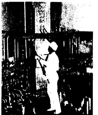
In Russia's Kola Nuclear Power Plant, a worker seals a confinement weld.
