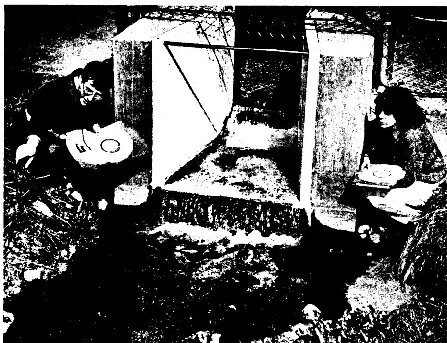
The Safety & Environmental Protection Division's Robert Lee and Barbara Royce inspect one of the new flow-monitoring stations located along the Peconic River, downstream of the BNL Sewage Treatment Plant.
