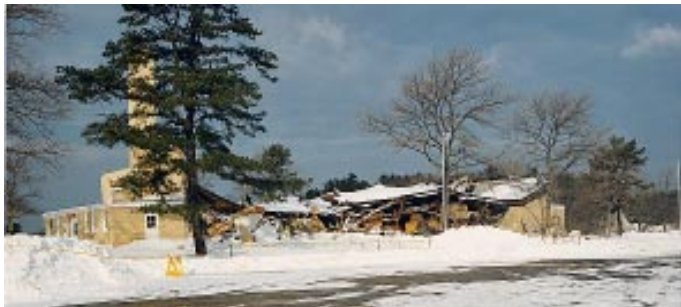
(above) Bldg. 424 in 1990. (below) The wreckage of Bldg. 424 after its complete collapse last January.
