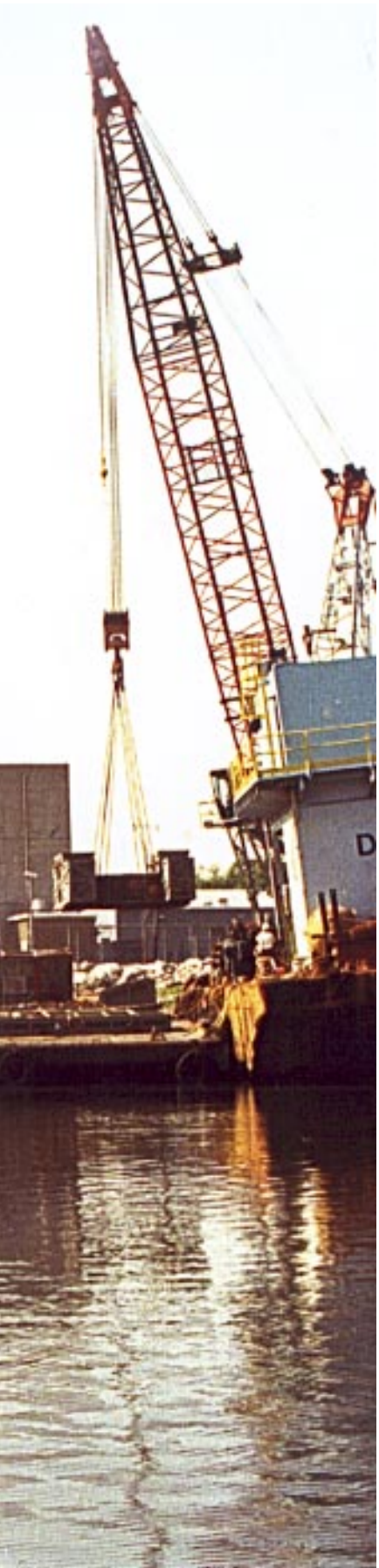
A crane hoists crates containing some of PHENIX's steel parts off a barge in Shoreham in early June. Nearly 2,600 tons of steel, some pieces as tall as 35 feet and as heavy as 100 tons, came to Long Island from Philadelphia on five barges after being shipped from St. Petersburg, Russia. The carefully shaped electromagnets and steel plates were made and machined in St. Petersburg's Izhora Steelworks, one of the few steel mills in the world capable of making such large objects, for PHENIX collaborators at the Petersburg Nuclear Physics Institute and the Efremov Institute for Electrophysical Research. The steel is now being installed in PHENIX's assembly hall, Bldg. 1008, located at the 8 o'clock position in the RHIC ring.
