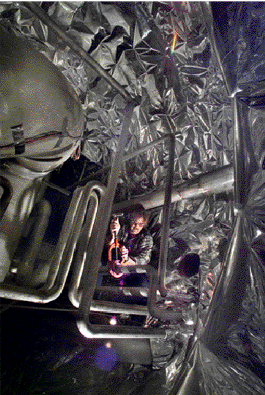
Surrounded by the superinsulation that protects the cold parts of the refrigerator from heat, Bill DeJong, Cryogenic System Section, prepares to install a new valve in some piping inside a cold box.
