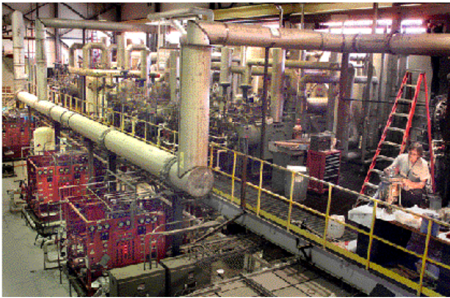
Inside the refrigerator building, Bill DeJong of the Cryogenic System Section inspects a turbine situated under the pipe linking the refrigerator to the two RHIC rings. The white containers (top, background) are cold boxes holding vacuum, piping and liquid-helium pots.
