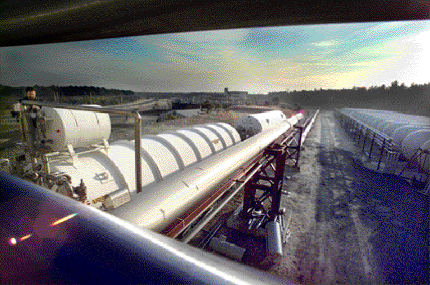
An overview taken of the liquid and gas storage area adjacent to Bldg. 1006B, where a Central Shops Division welder (left) stands near one of the three 11,000-gallon helium dewar tanks. Further back lies a liquid nitrogen tank, and at right are the helium-gas storage tanks. The superinsulated dewars maintain the liquid and gas inventory at approximately 4.6 Kelvin (-269°C).
