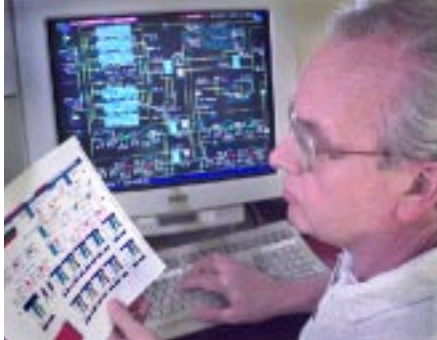
In the control room, Dieter Zantopp of the Cryogenic System Section reviews a page of cryogenic control systems. On the screen is a typical control page, which the Cryo group uses to operate the 25-kilowatt refrigerator. By the push of a button, a 2,000 horsepower motor, or turbines, or any piece of process equipment can be started or shut off. The control system is also used to identify system faults and automatically maintain process control.
