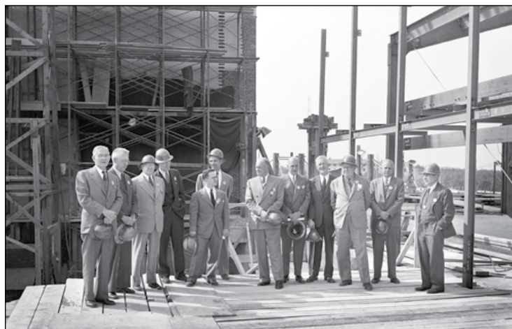
In October 1948, the BGRR construction site was toured by (from left), George Pegram, Columbia University; Harold Dodd, president of Princeton University; Frank Fackenthal, Columbia; either* Karl Hartzell, Associated Universities, Inc., or* Henry Smyth, Princeton; David Gurinsky, BNL; Leland Haworth, BNL Director; Dwight Eisenhower, president of Columbia; Charles Seymour, president of Yale University; William Watson, Yale; George Brakeley, Princeton; Edmund Sinnott, Yale; and Isidor I. Rabi, Columbia. *Any thoughts on this ID problem? Contact lseubert@bnl.gov , Ext. 2346.
