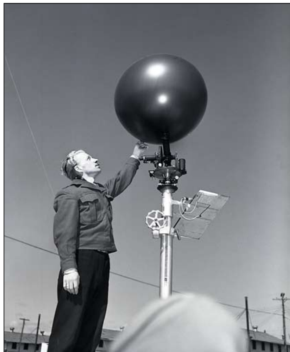
In April 1948, technician Frank Scott is releasing a pilot balloon, which will have its flight checked in the "theodolite" device to determine wind conditions.
