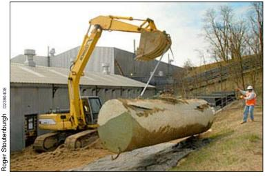
On April 8, BNL marked a major milestone in its ongoing efforts to protect the environment when the last single-walled underground storage tank on the property was excavated and sent off site for recycling. The 3,000-gallon tank used to store diesel fuel was in good condition and had never leaked. It did not, however, meet today's stringent codes for underground fuel-oil storage in Suffolk County.
