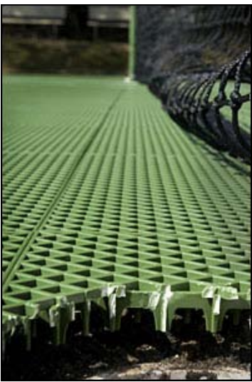
The new court flooring is raised off the surface to facilitate drainage and prevent water damage.
