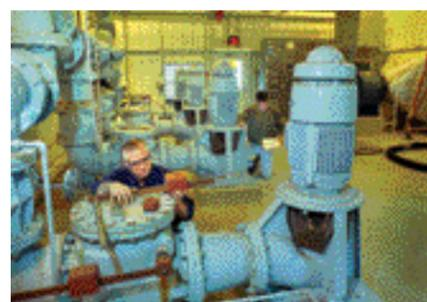
air-stripping towers. Viewed in the wet-well pump room, Richard Lutz (front) works on a check valve, while Jack Kulesa inspects pump seals.
