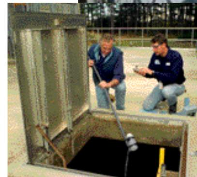
**STEP 10.** At the clear well, where up to 250,000 gallons of “finished” water is stored before its final chlorination and distribution, Richard Lutz (left) and Jack Kulesa take samples.
