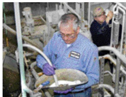
**STEP 5.** Polymer is added to aid in flocculation (see step 6). Richard Lutz (front) is seen adding polymer into a rapid-mix tank, as Phil Pizzo adjusts the flow rate.
