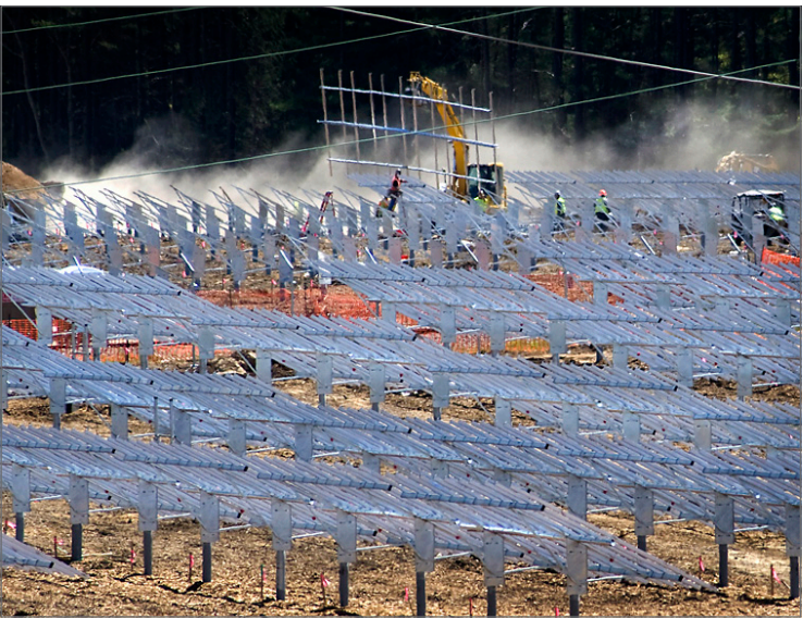
Racks in place to hold thousands of solar panels at the LI Solar Farm at BNL
