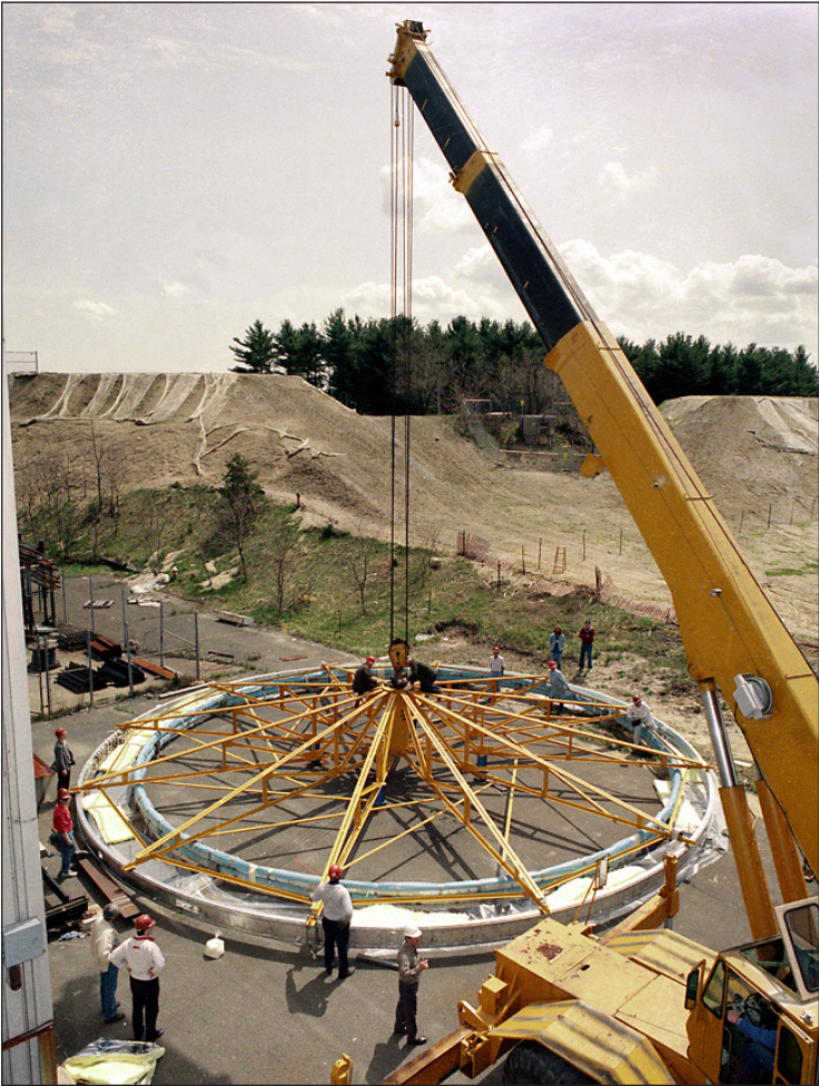
Got the Coil on a String! In April 1992, as the Bulletin reported, the world's largest superconducting coil “on a string” was hanging not from a finger but from a massive crane outside Bldg. 919. Three coils had been constructed inside the building. The third and largest coil was pulled on special heavy-duty tracks past a removable wall to the outdoors, attached to the crane, then lowered into its final position on the foundation that held the two previously completed inner coils within the building. Work then continued to ready the experiment for the storage ring’s commissioning scheduled for December 1993.
