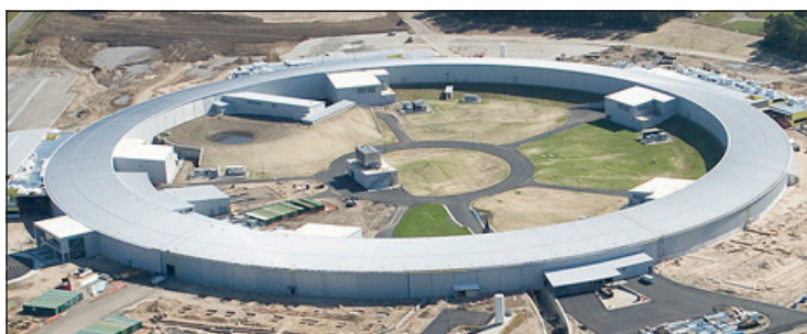
This Linac will be the electron source for NSLS-II: a new state-of-the-art, medium-energy electron storage ring (3 billion electron-volts) designed to deliver world-leading intensity and brightness, and produce x-rays more than 10,000 times brighter than the current NSLS. NSLS-II is on track to begin operations in 2015.
