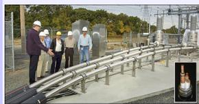
LIPA commissioned the 1st high temperature superconducting power transmission cable (138 kV) system on June 25, 2008 at Holbrook site, Long Island, NY, capable of carrying 574 megawatts of power.
