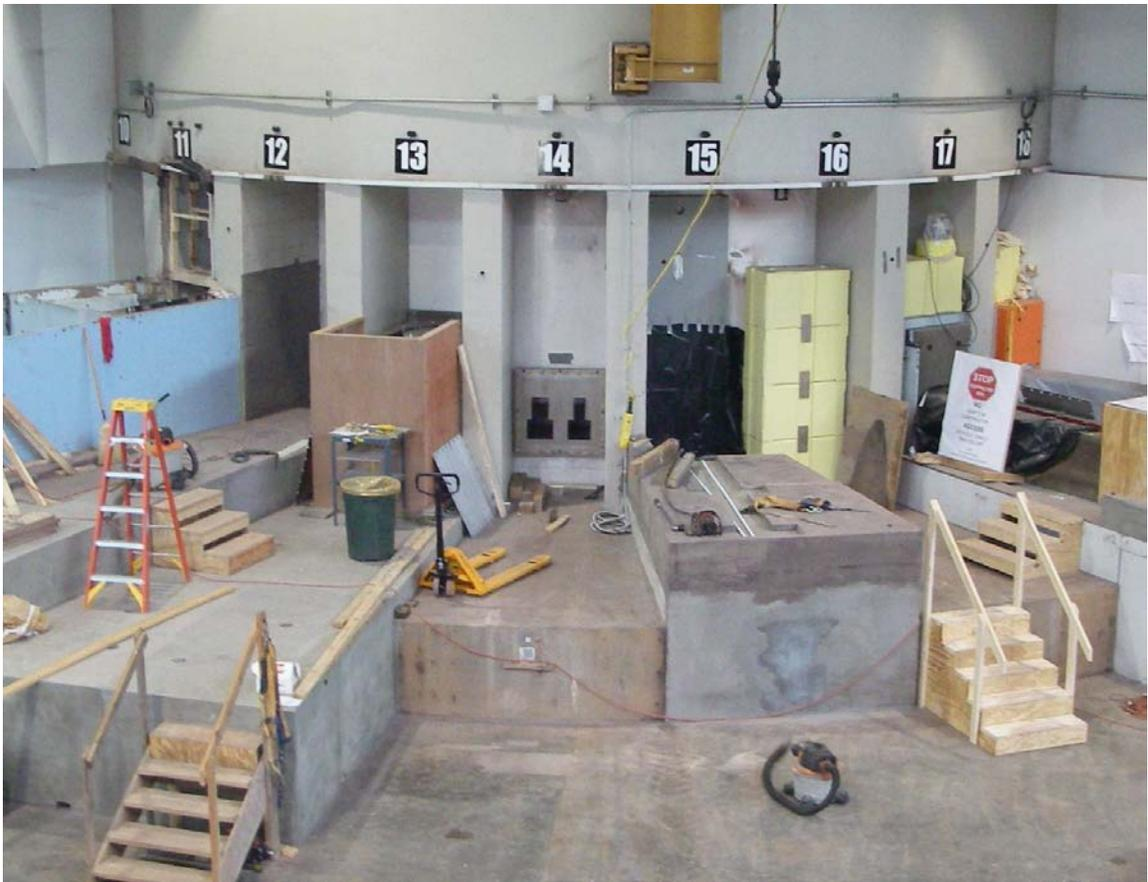
Bulk Shield Insert in place in HYSPEC (14) Beamline
