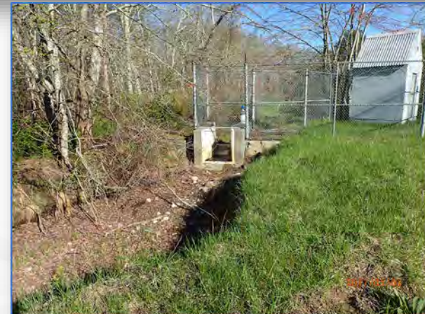
Monitoring Station HM-N
