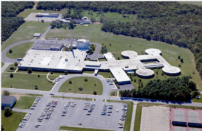
Building 490 – former Medical Complex
