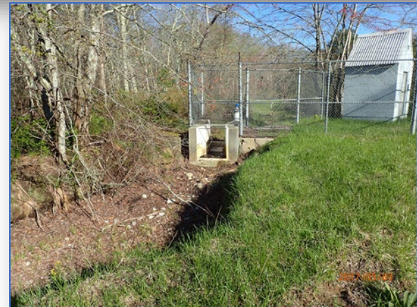
Monitoring Station HM-N
