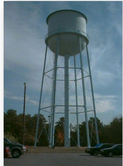
WW II era Water Tower
