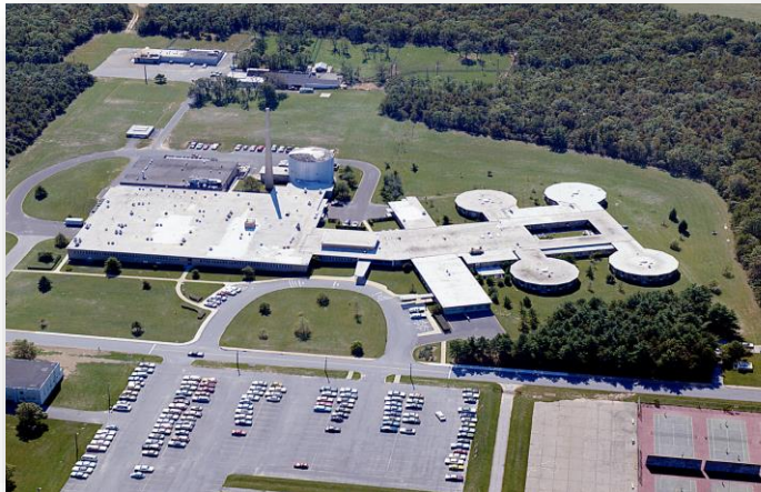
Building 490 – former Medical Complex
