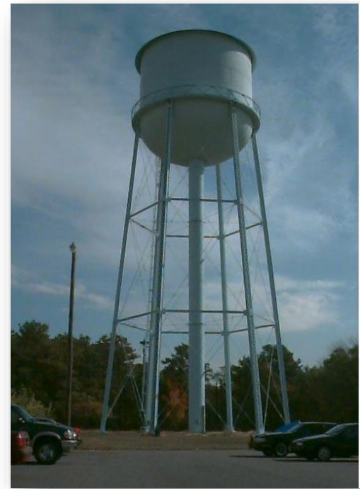
WW II era Water Tower
