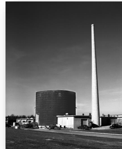
BMRR w/stack c. 1958
