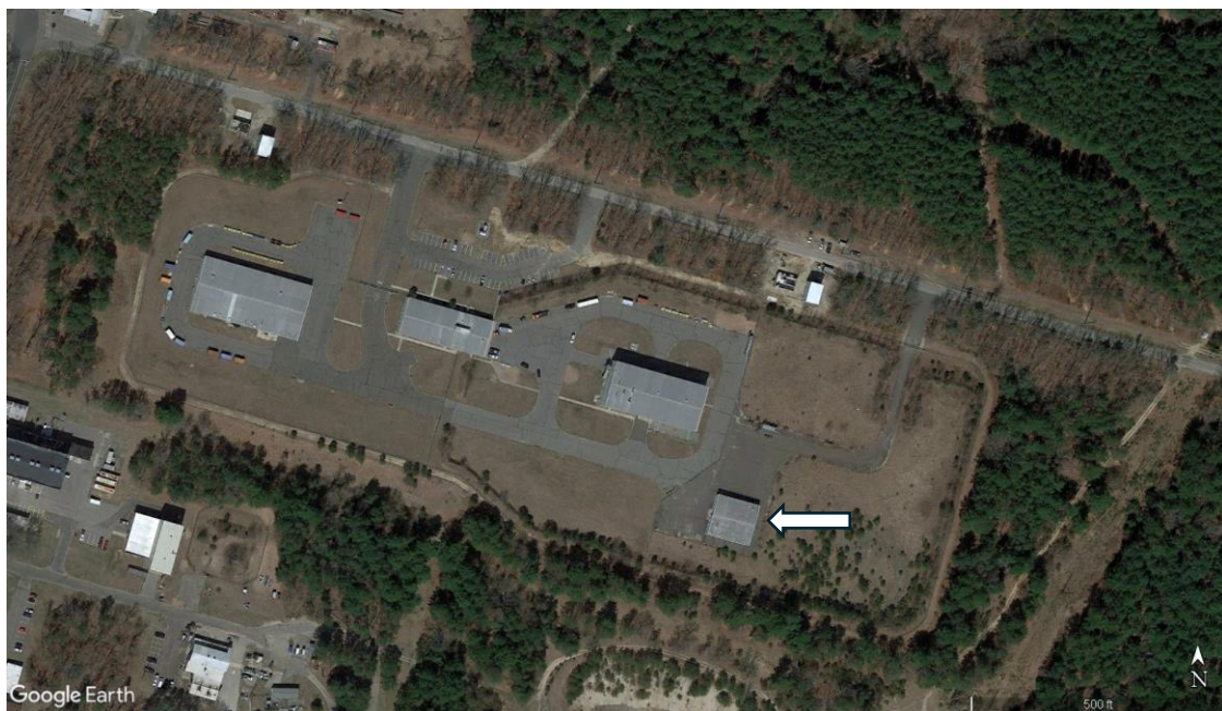
Waste Management Complex, building 870 (left-center at arrow).
