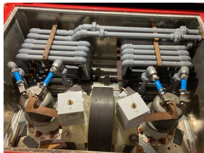
Booster Main Magnet Cooling System piping – after replacement
