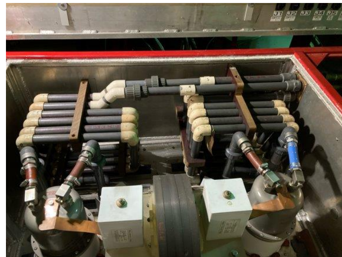
Booster Main Magnet Cooling System piping – before replacement
