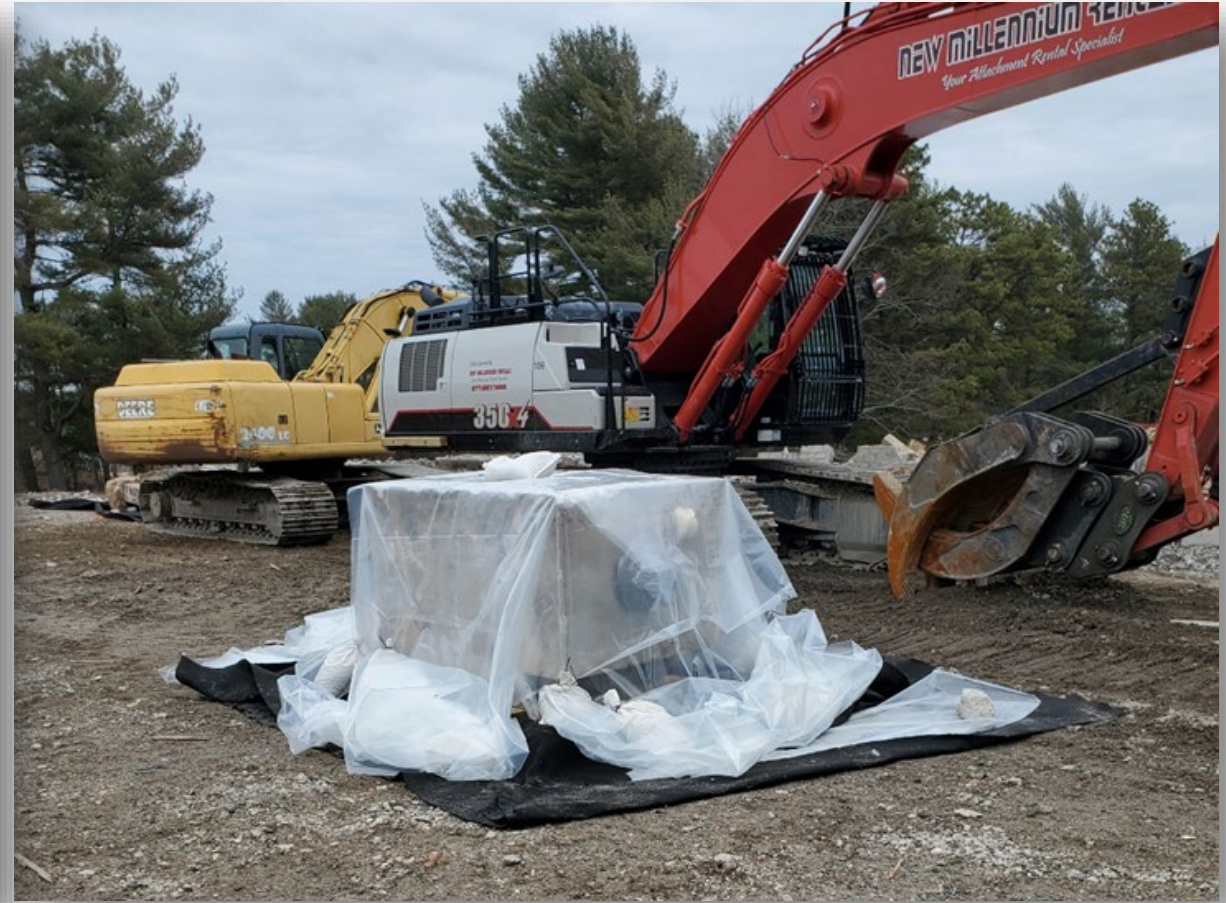
Concrete structure containing elemental mercury in a secondary containment pad
