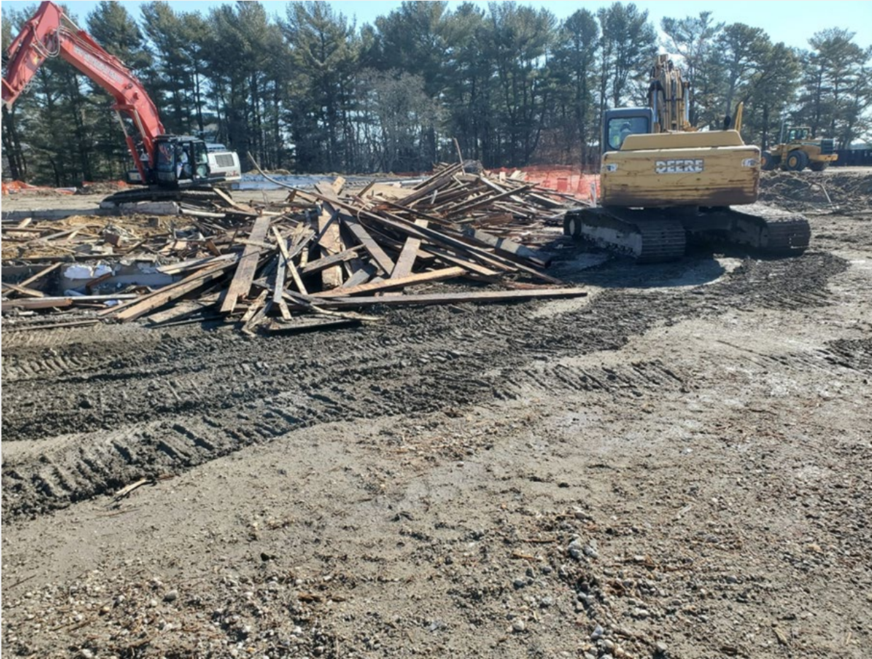
Wood floor removal in process
