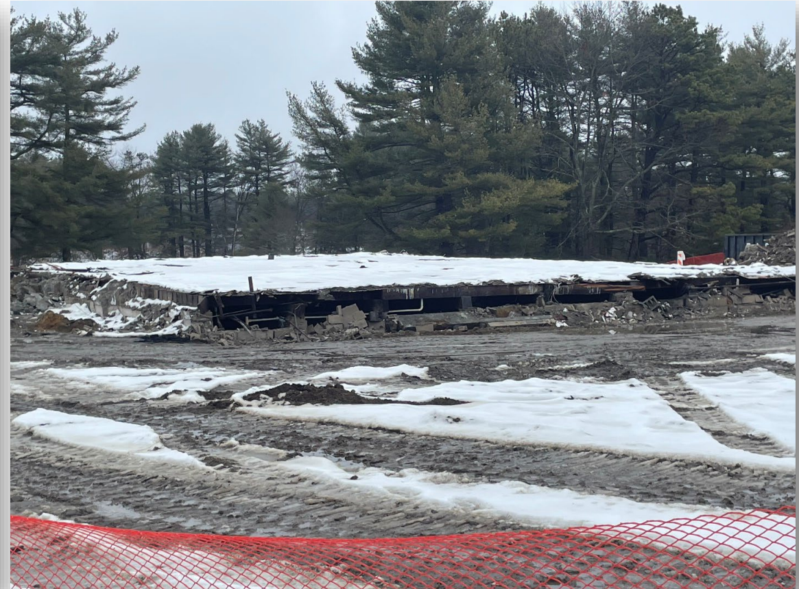
Demolition progress of the building 2/13/25. The wood deck is cleared off and the outside wall on the foundation was removed
