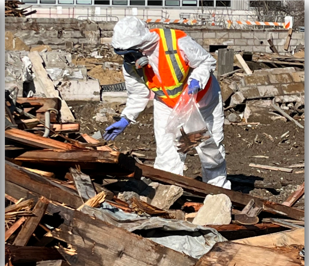
Sampling of wood floor for waste characterization purposes
