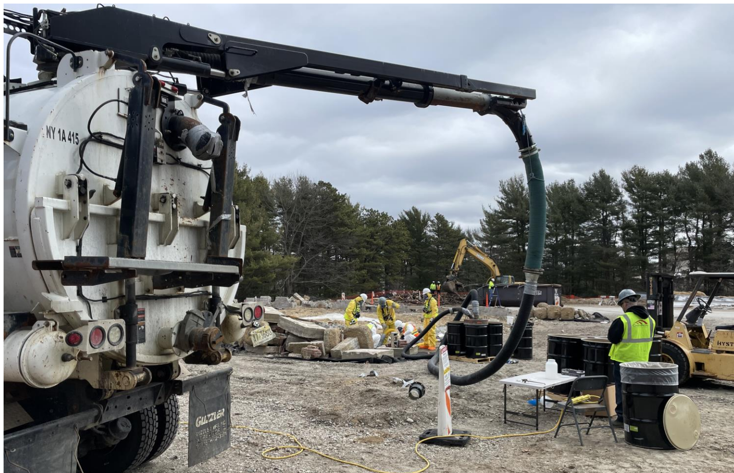
Crew working on west side of building footprint removing soil/elemental mercury mixture using vacuum guzzler.
