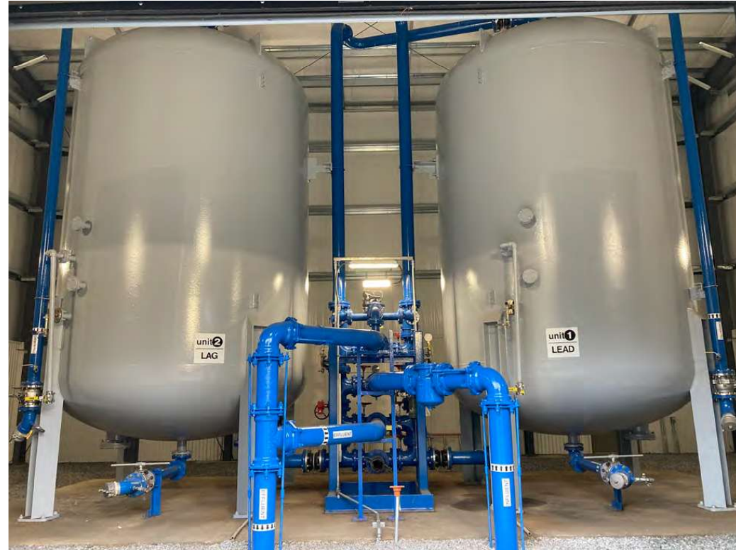
Treatment System for Former Firehouse PFAS Plume Granular Activated Carbon Filters
