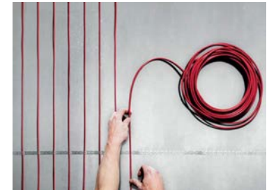
Resistance wiring
