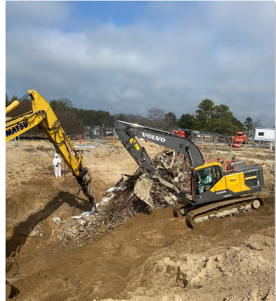
View of the silencer demolition process looking from the south
