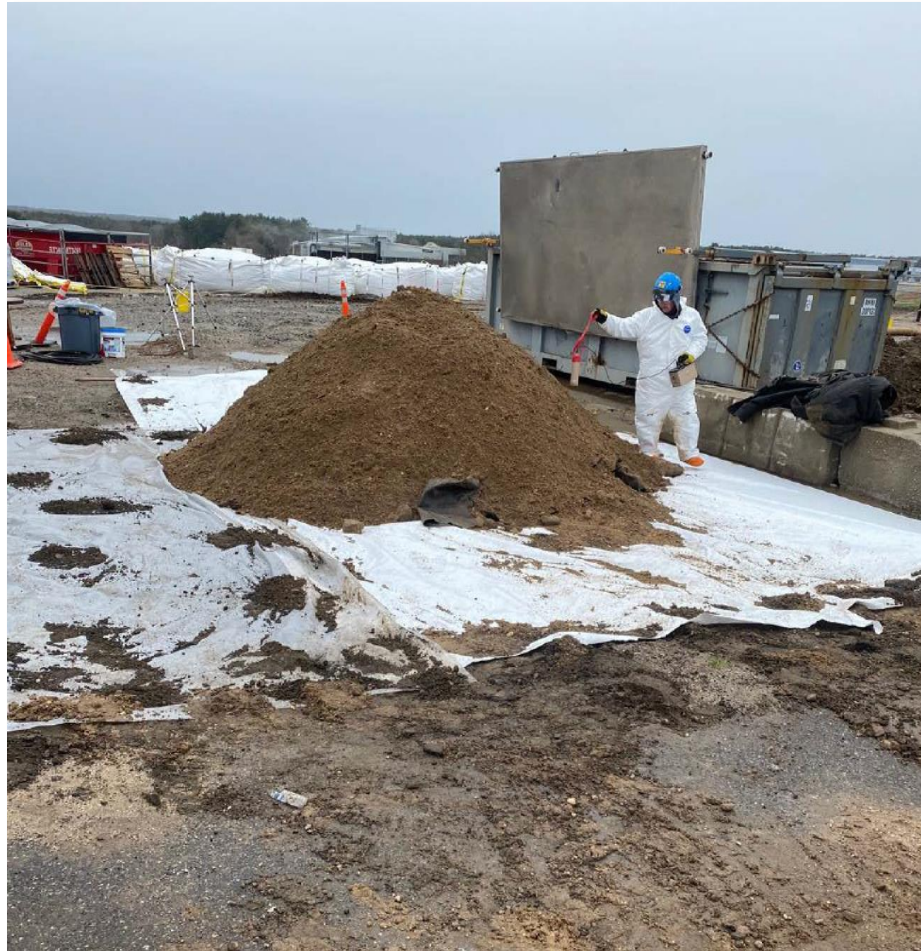
Initial rad screening of stack drain tank overburden soil
