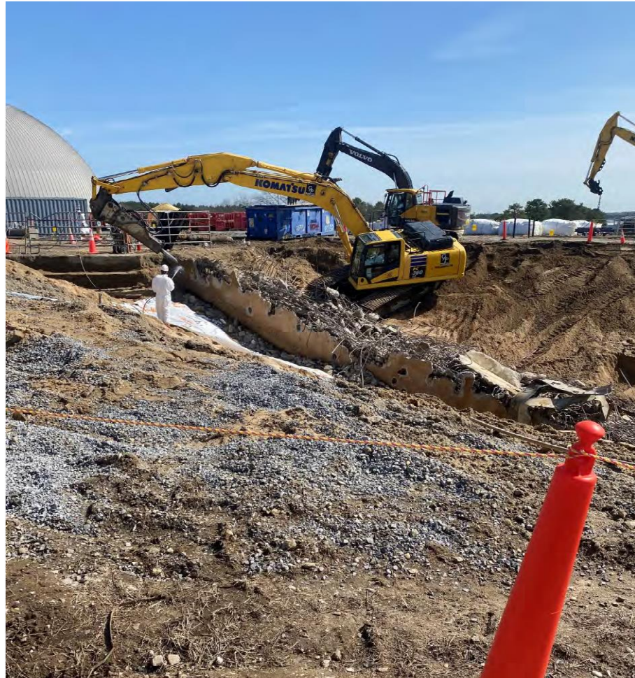
View of silencer demolition from the north
