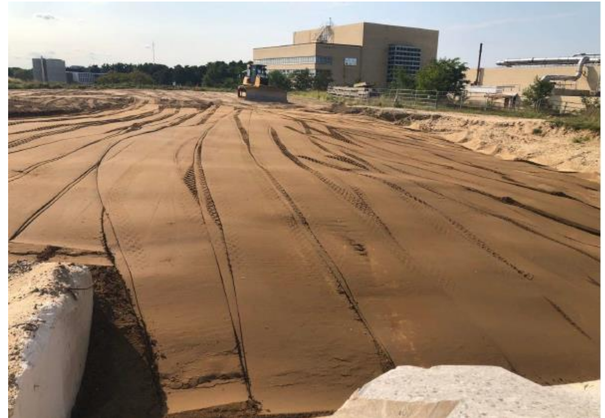
View looking northwest at the silencer excavation area backfilled and compacted (SEP21).
