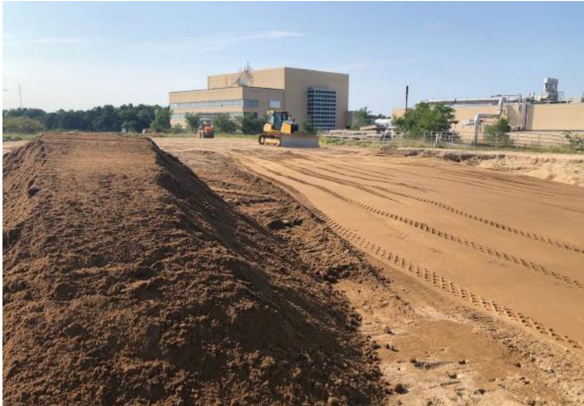
View looking northwest at the silencer excavation area backfilled and compacted (SEP21).
