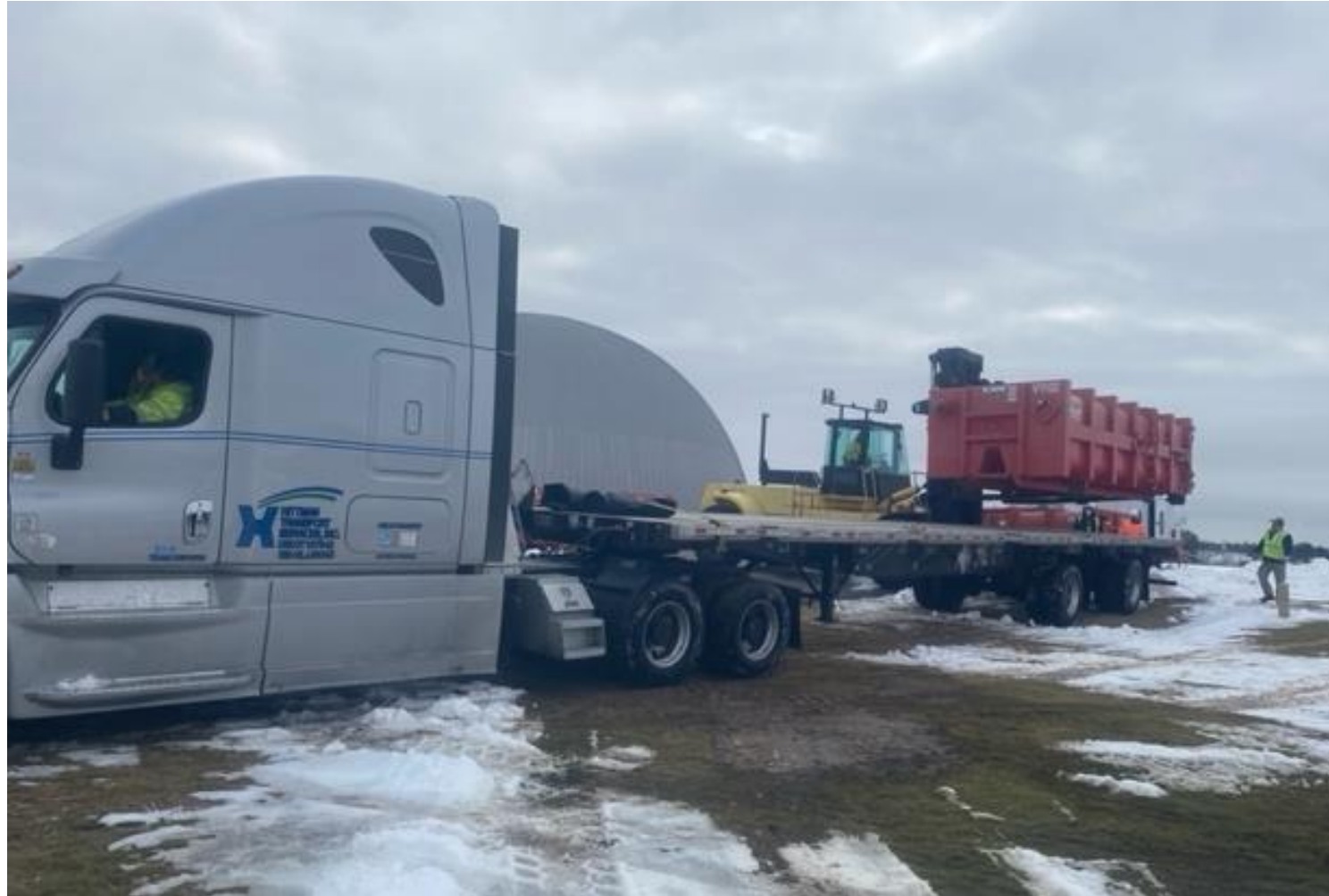
Wastewater tanks being removed off site (FEB22).
