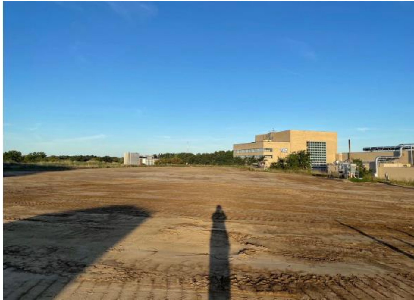
Completion of backfill and compaction looking west (SEP21).
