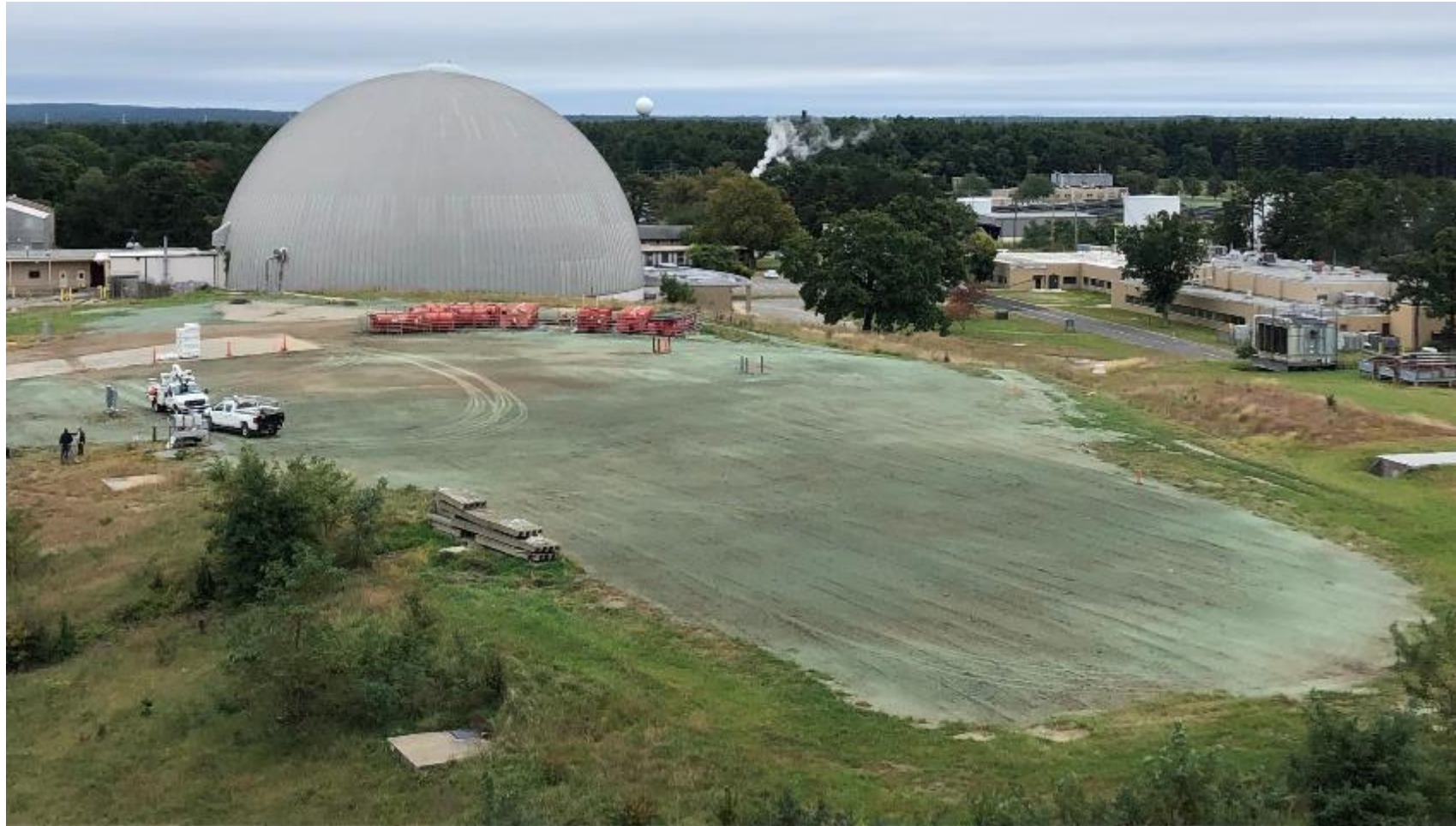
Hydroseeding looking east (OCT21).
