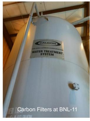
In the 1980's, carbon filters were installed on three supply wells to remove VOCs. They were taken out of service ~10 years ago
