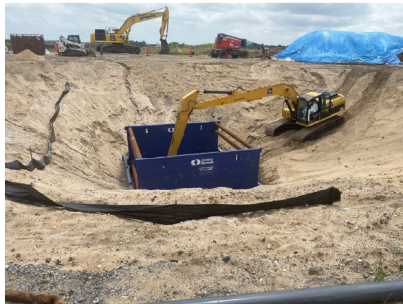
HFBR stack area soil excavation 2021
