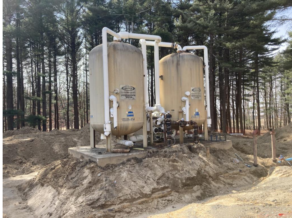
Preparing for Construction of Former Firehouse GAC Filter System Building
