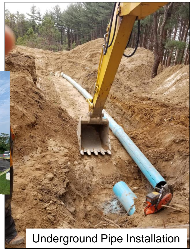
Extraction Well Installation South of Former Firehouse Area
