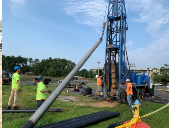
Extraction Well Installation South of Former Firehouse Area
