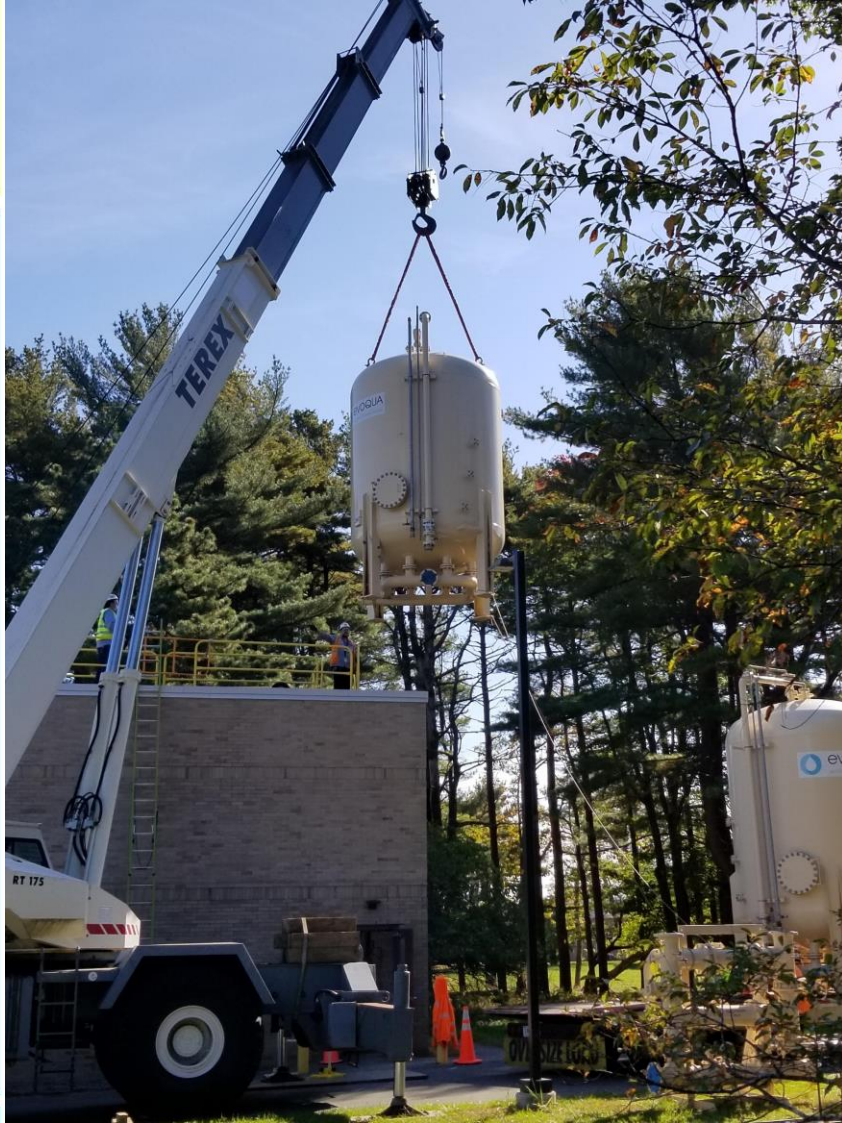
Installing GAC Filters at Current Firehouse Treatment System Building
