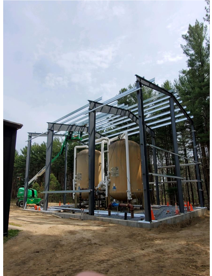
Construction of Former Firehouse GAC Filter System Building
