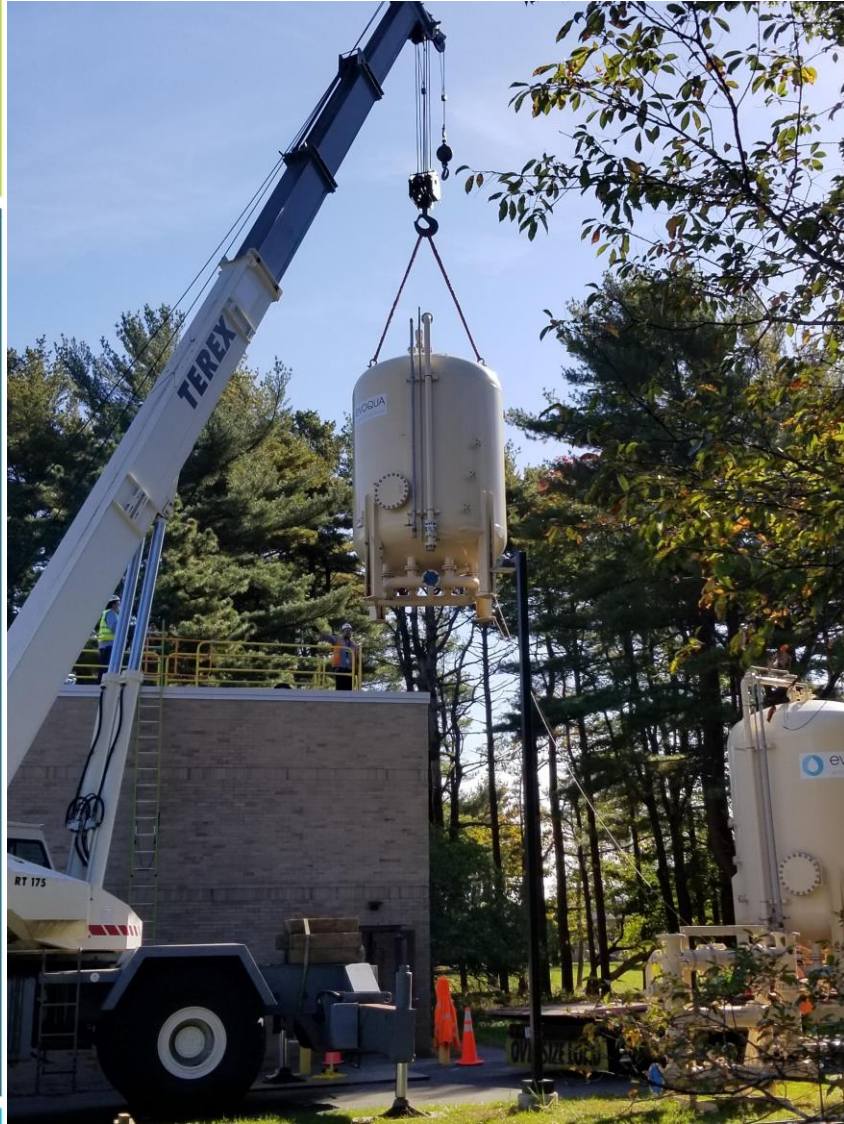
Installing GAC Filters at Current Firehouse/Building 170 Treatment System Building
