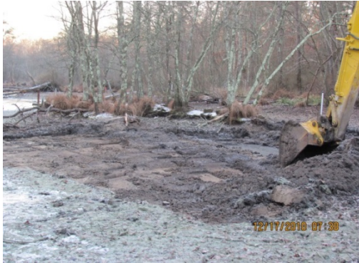
12/2010 looking downstream Area 6 during cleanup
