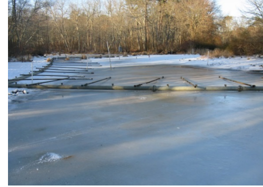
1/2011 well points for dewatering just prior to excavation looking upstream
