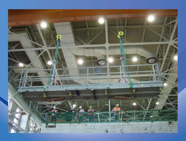
Three balconies attached to the pile had to be removed to install the cranes and CCE
