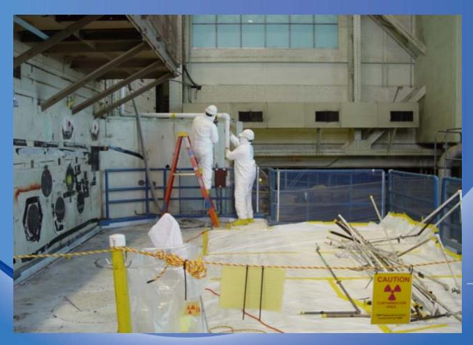
Numerous conduits and service piping were removed for CCE installation
