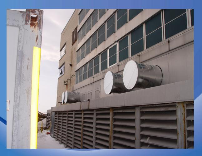
HEPA ventilation exhausts ducts waiting to be connected to blower trailer
