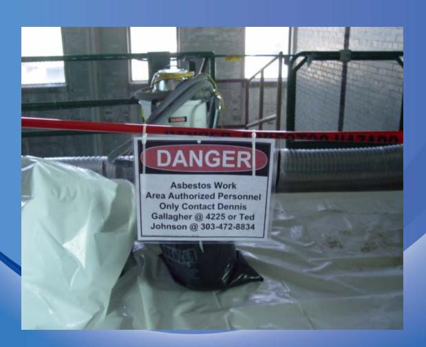
Asbestos containing floor tiles were removed from all elevations in contact with the graphite pile
