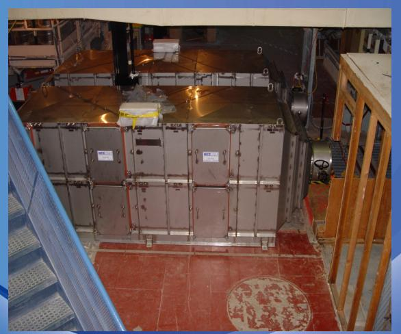
One of the four HEPA units being installed to provide filtration of radioactive airborne particulates during graphite pile removal
