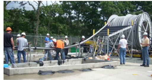
The LIPA-DOE Holbrook Superconductor Project: 600-m long cable, powers 300,000 homes, needs 13,000 gallons of LN 2
