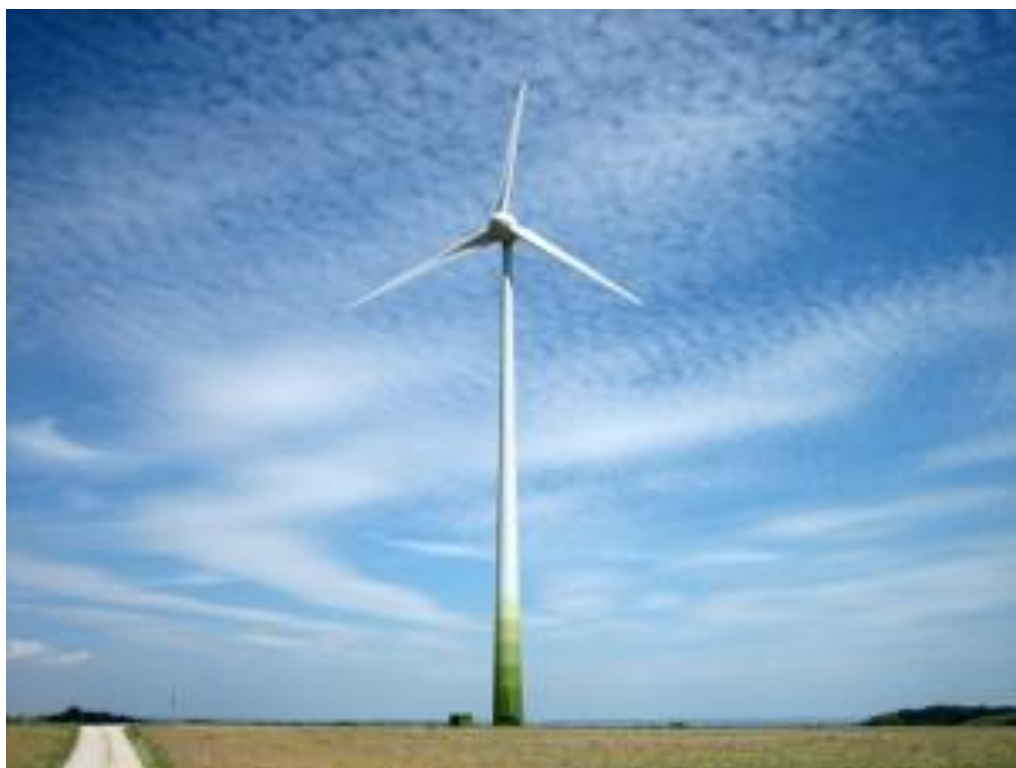
(Above) Enercon E53 500 kW wind turbine. Source: http://www.renewablesfirst.co.uk/windpower-wind-turbines/
