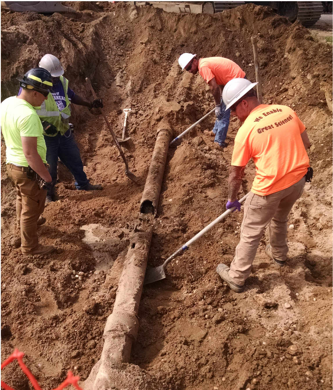
Figure 1. A main break at BNL in the summer of 2019. These happen frequently onsite which is why it's important to know how to properly handle them.
