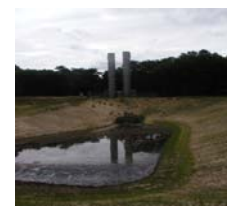
Fig. 7 P-16 Recharge Basin
