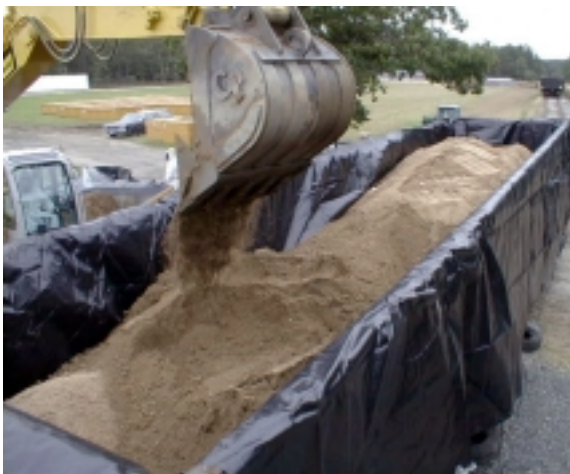
Figure 4-3. Railcar Loading of Contaminated Landscape Soil.
