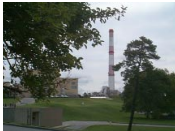
Figure 4-3. HFBR and Evaporator Facility Exhaust Stack.
