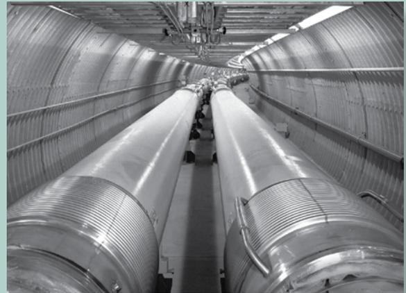
BNL's Relativistic Heavy Ion Collider has two accelerators in one made of crisscrossing rings of superconducting magnets enclosed in a tunnel 2.4 miles in circumference. In the two rings, beams of heavy ions are accelerated to nearly the speed of light in opposite directions, held in their orbits by powerful magnetic fields.
