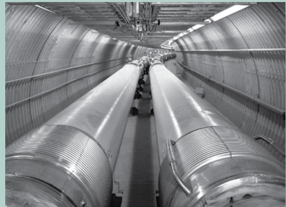
BNL's Relativistic Heavy Ion Collider has two accelerators in one made of crisscrossing rings of superconducting magnets enclosed in a tunnel 2.4 miles in circumference. In the two rings, beams of heavy ions are accelerated to nearly the speed of light in opposite directions, held in their orbits by powerful magnetic fields.
