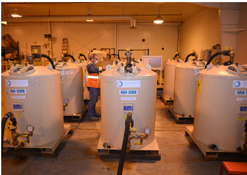
Brookhaven Graphite Research Reactor Sr-90 Groundwater Remediation System Ion-Exchange vessels.
