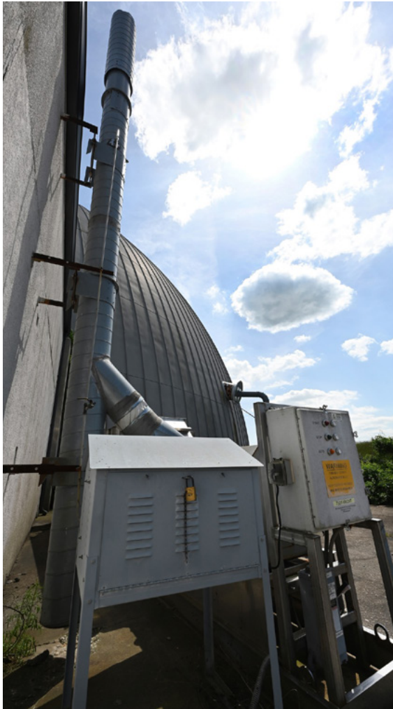
Sampling station for airborne tritium in the HFBR building exhaust.
