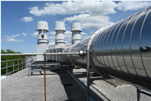
Emissions sampling point for exhaust from the Radionuclide Research and Production Laboratory (RRPL) (stacks in background).
