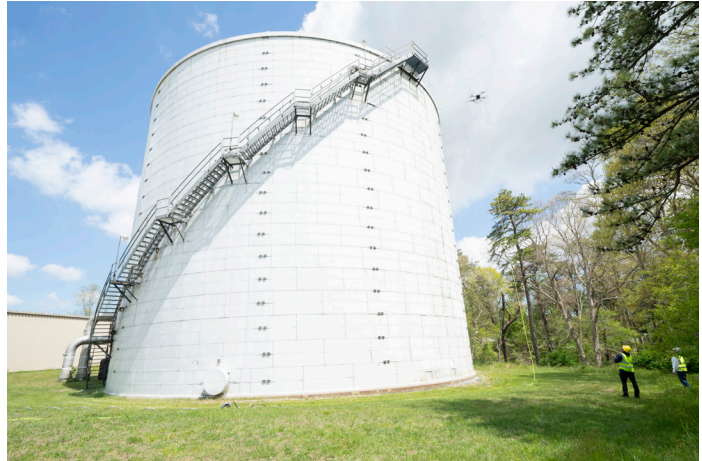
BNL's 3.2 million gallon chilled water storage tank used to reduce peak electric demand by producing and storing chilled water is getting cleaned remotely, via drone.
