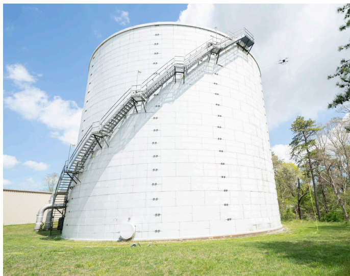
BNL's 3.2 million gallon chilled water storage tank used to reduce peak electric demand by producing and storing chilled water is getting cleaned remotely, via drone.
