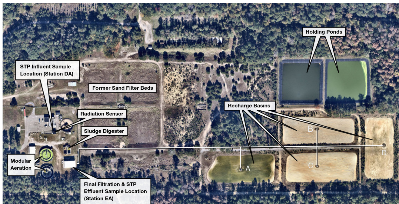
Figure 4-1. An aerial photo of BNL's Sewage Treatment Plant (Recharge Basin Discharge)
