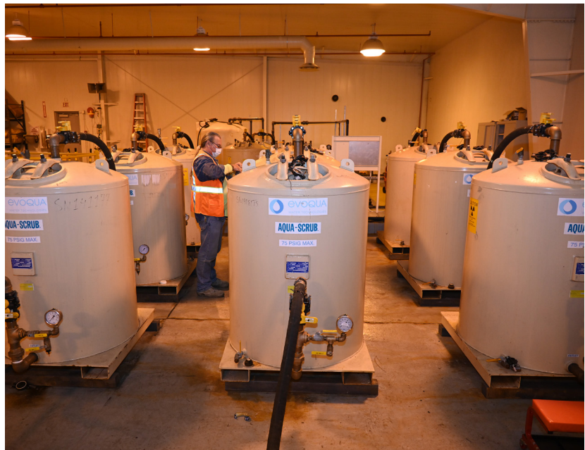
Brookhaven Graphite Research Reactor Sr-90 Groundwater Remediation System Ion-Exchange vessels.
