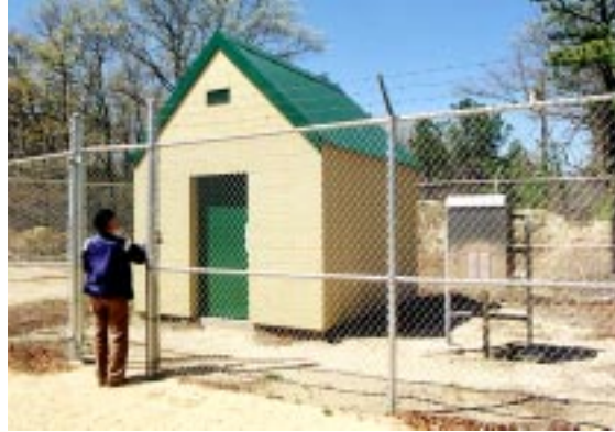
Figure 5-3. Environmental Air Sampling Blockhouse
