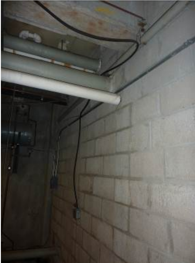
Picture C7. Does not comply with 400.8(1). The flexible cord is used as permanent wiring.
