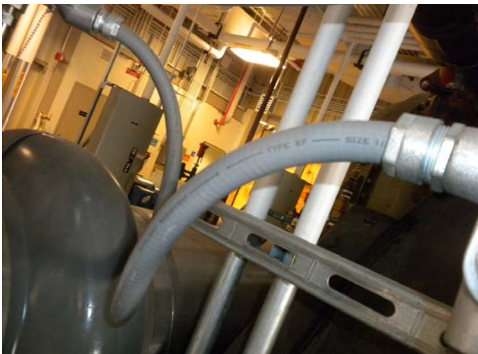
Picture B1. Liquidtight Flexible Metal Conduit does not comply with NEC 350.6 since it is not listed by NRTL.
