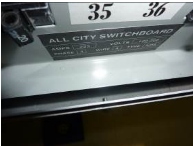
Picture C8. Does not comply with 110.3(B). Modifications of panelboard invalidates UL
