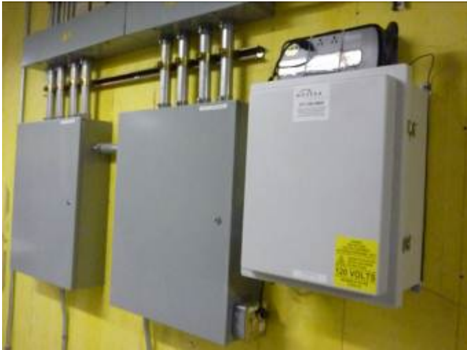
Picture A5. Conduit compliantly supported.
