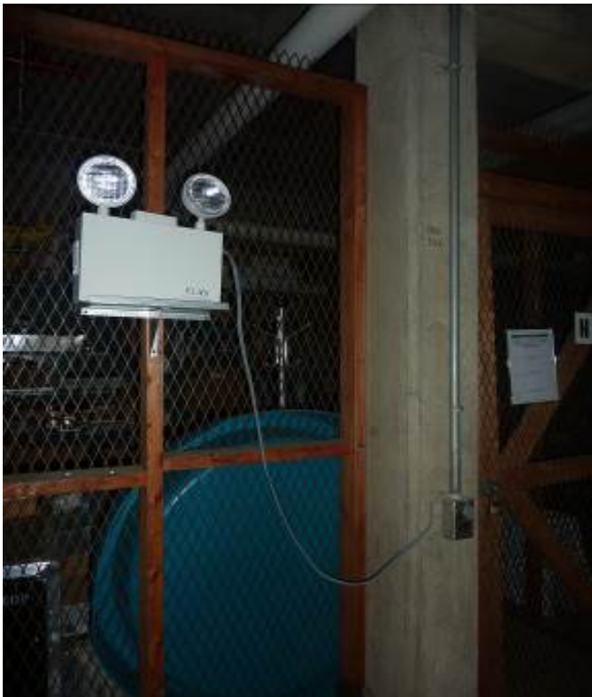
Picture C2. Does not comply with 700.12(F). Emergency unit not connected to lighting circuit ahead of switch and power cord exceeds 3' length.
