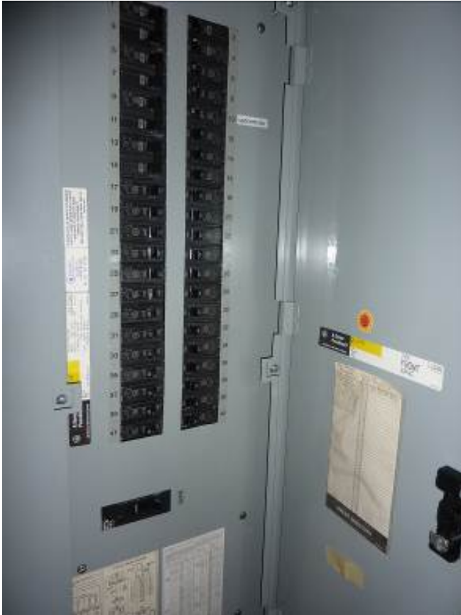
Picture C3. Does not comply with 408.4. Panel schedule not complete.
