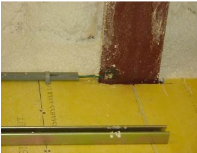
Picture A4. Proper grounding of Separately Derived System.
