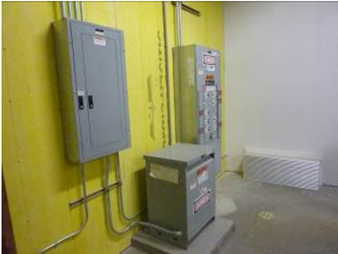
Picture A3. Working clearance observed.
