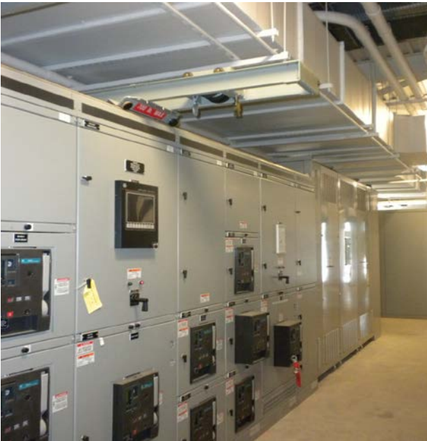
Picture B5. Does not comply with NEC 110.26(F)(1). Duct within the dedicated space of switchboard.
