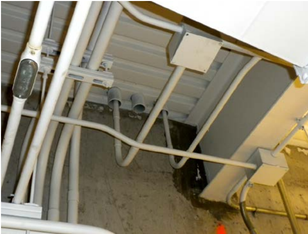
Picture B4. Does not comply with NEC 344.23(B)(1). Rigid Metallic Raceway not supported at 10' intervals and within 3' of an enclosure.
