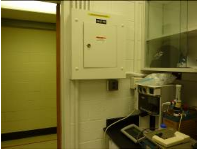
Picture C9. Does not comply with 110.26(A). Added counter encroaches on working space.
