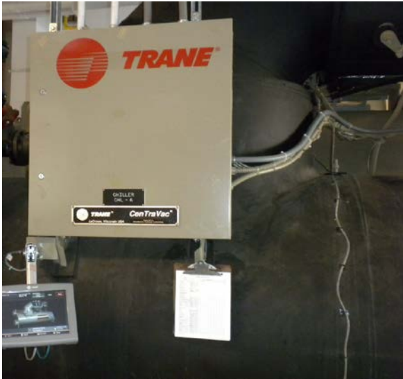
Picture B2. Does not comply with NEC 300.11(B) and 350.30. Raceway supporting other cables and conduit not supported within 12" of box.
