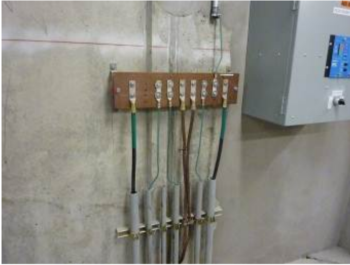
Picture A1. Proper grounding and bonding of the electrical distribution system.
