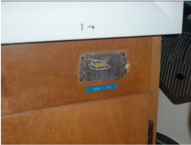
Picture C1. Electrical equipment not approved and does not meet requirements of 110.3(A) for suitability.
