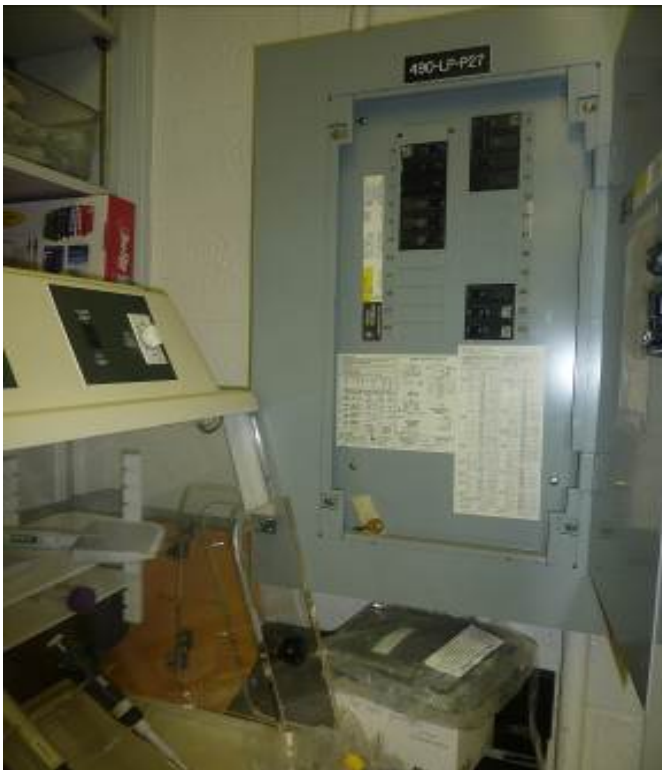
Picture C6. Does not comply with 110.26(A). New panelboard installed without working space.
