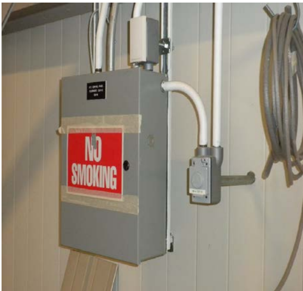
Picture B3. Does not comply with NEC 314.23(F). Raceways supporting enclosure not secured within 18".
