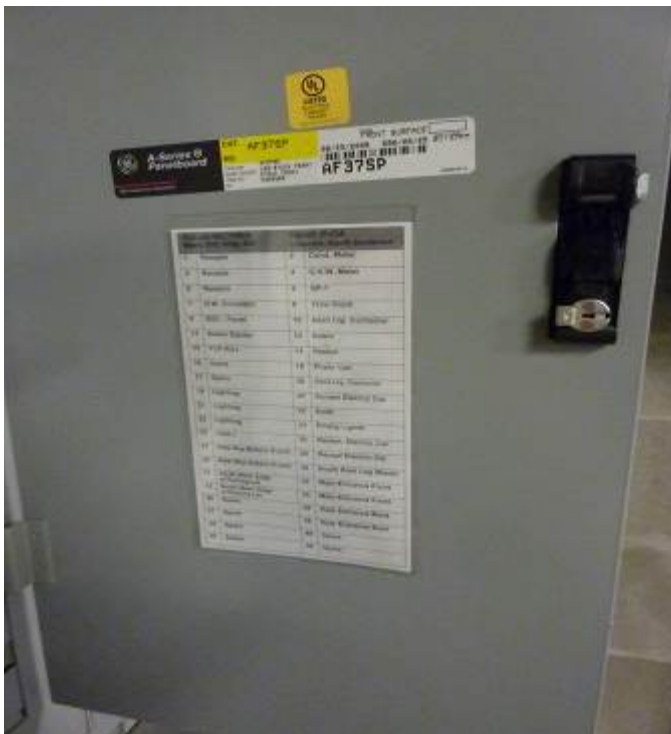
Picture A2. Panel schedule complete and accurate.
