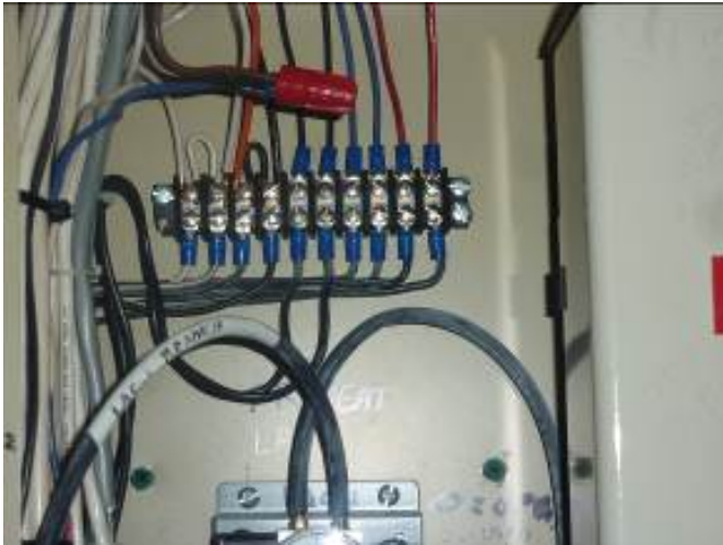
Picture C5. Does not comply with 110.27. Energized conductors are not adequately guarded.
