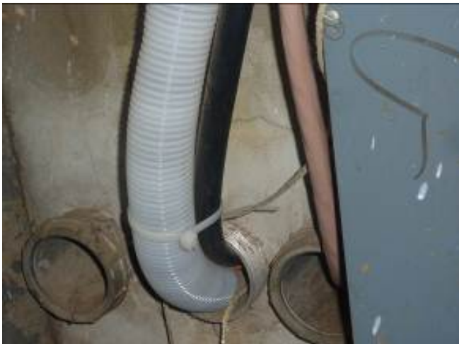
Picture C4. Does not comply with 400.8(2). Flexible cord routed through wall.
