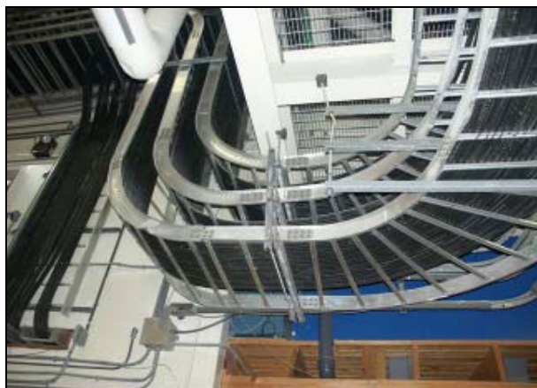
Figure 1 – Proper Cable Tray Installation
