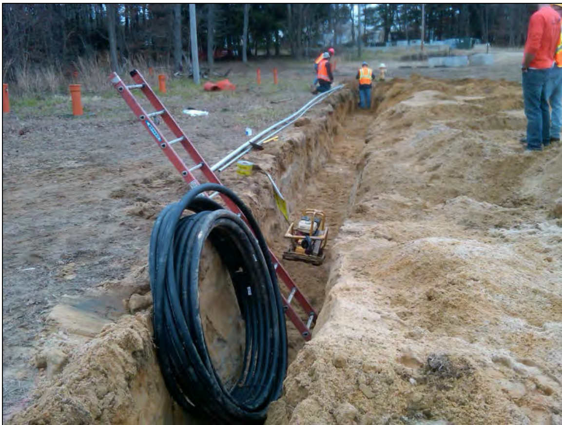
Figure 4. Installation of water, electrical and communications lines between extraction well EW-18 and the Freon-11 groundwater treatment shed.
