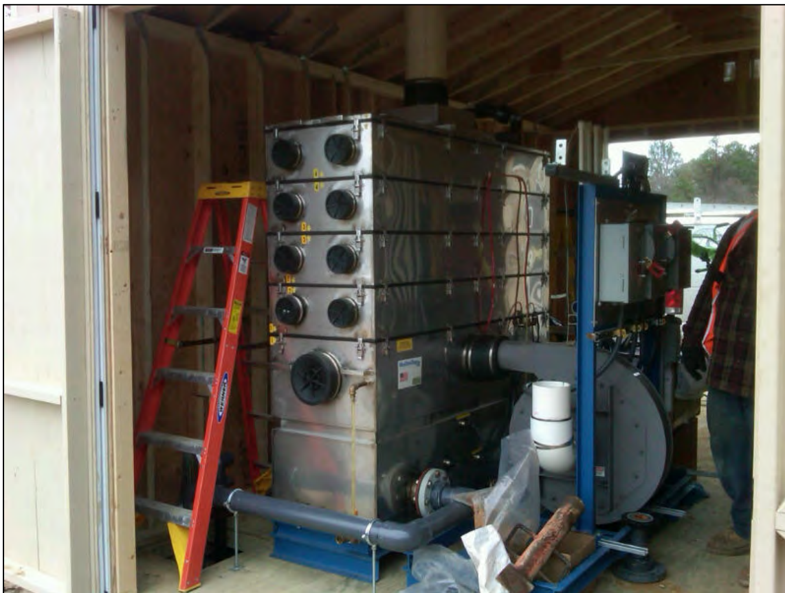
Figure 5. Installation of the air stripper trays in the Freon-11 treatment shed.
